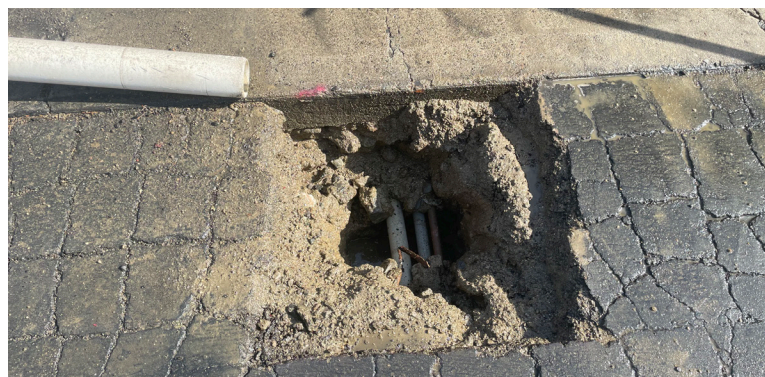
Crews working on utility line location work.
