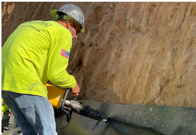
Crews installing waterproofing material for the retaining wall support system.
