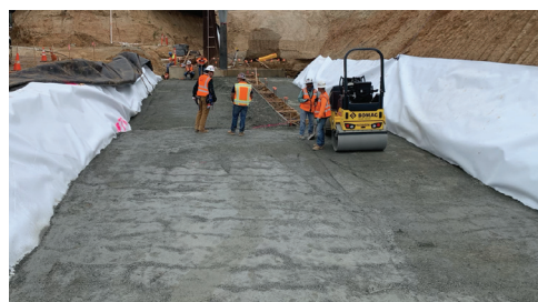
Crews continue to install geomembrane, a material that provides a moisture barrier, and cement treated base for the retaining wall structure foundation for the Jurupa Road underpass support system.
