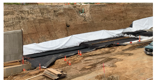
Crews continue to install geomembrane, a material that provides a moisture barrier, and cement treated base for the retaining wall structure foundation for the Jurupa Road underpass support system.
