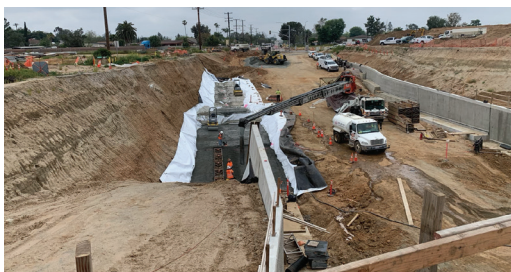
Crews continue to install geomembrane, a material that provides a moisture barrier, and cement treated base for the retaining wall structure foundation for the Jurupa Road underpass support system.
